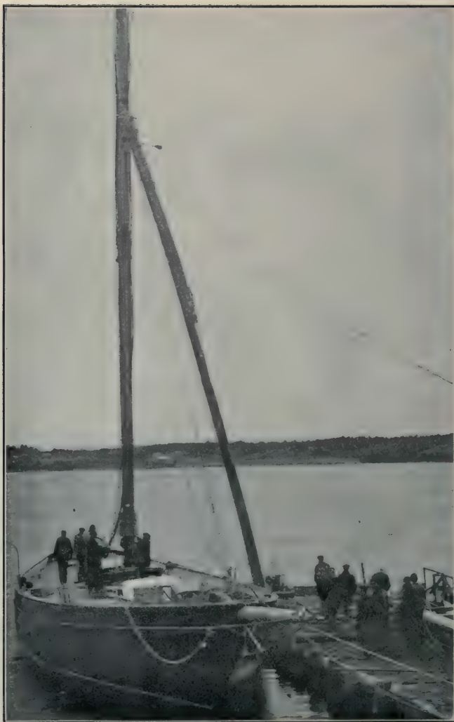
PLACING A MAST IN A SAILING VESSEL
